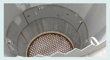
Actina™ reduces calcium hardness, metals, organics and other contaminants with a simple, fluidized bed reactor that uses a catalyst (sand, pellets) to promote calcium carbonate precipitation. A strainer plate is located at the bottom of the reactor and is specifically designed for pellet softening that allows for material in raw water to pass. Caustic/lime plus softened carrier water is pumped to a removable chemical dispersion unit for pH adjustment.
